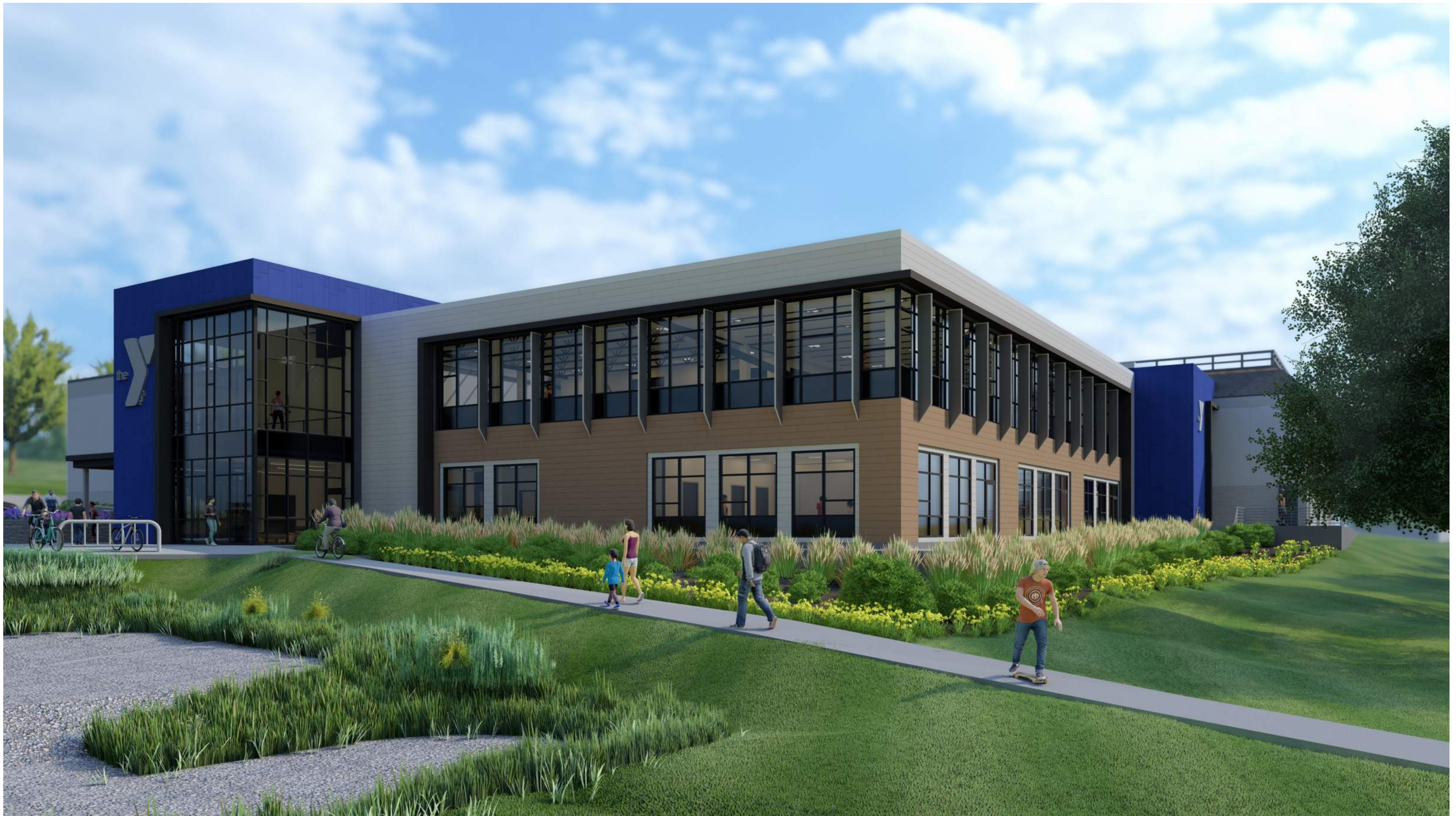
VIEW FROM ENTRANCE DRIVE
